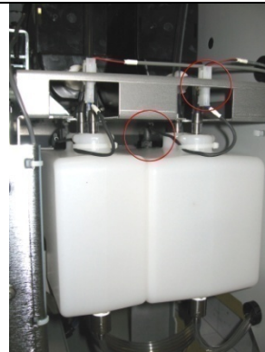
Binder bottle float switch and connector Figure 6
